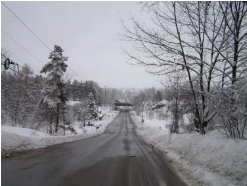
Looking East at I-89 Overpass on Crosstown Road
