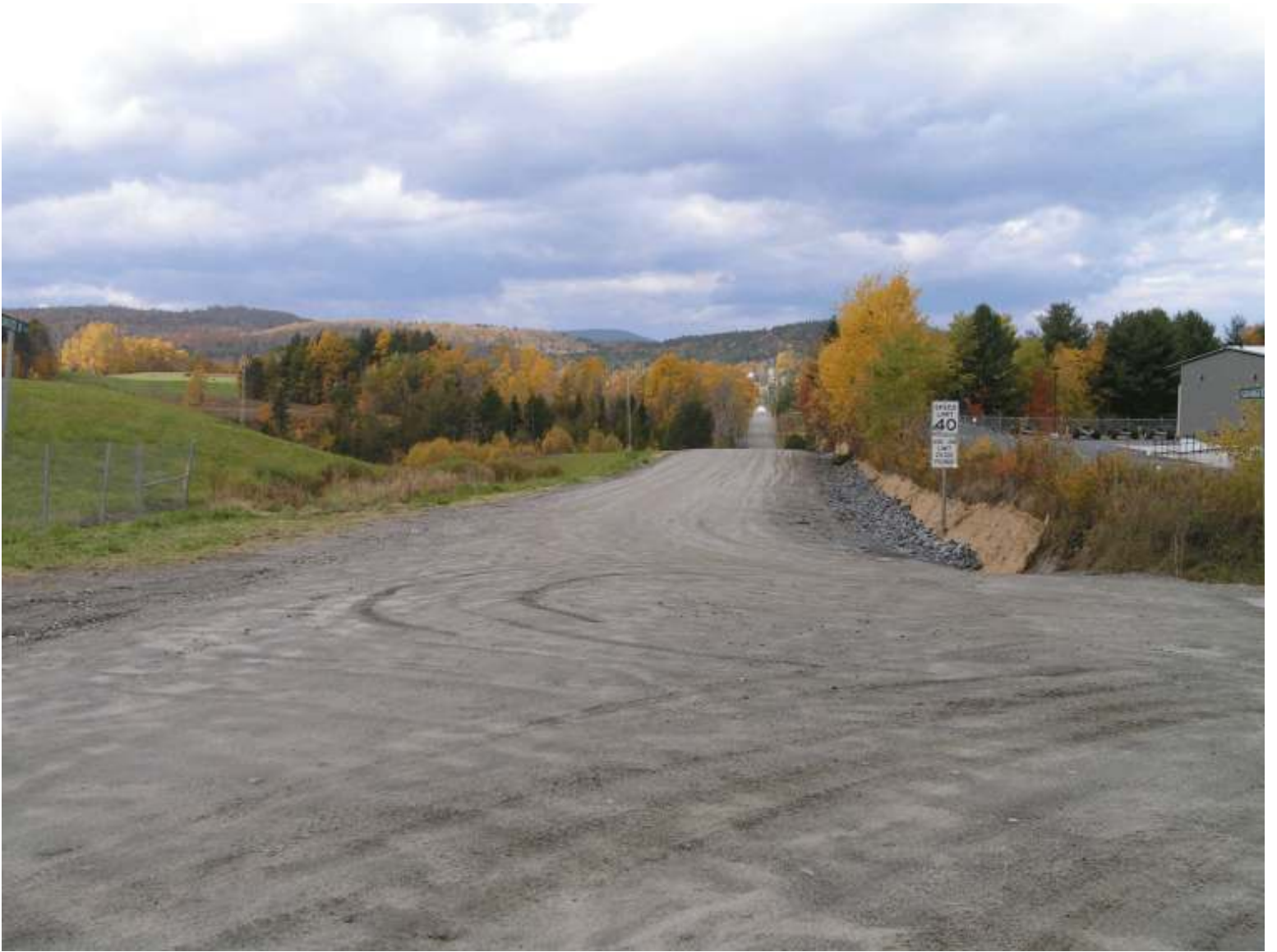
Comstock Road at its intersection with Granger Road looking West The Knapp Airport is to the left
